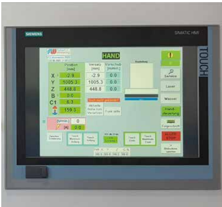
Bedienpanel, control panel
